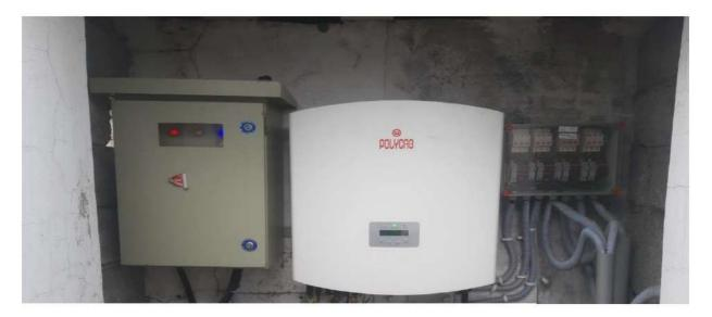
3. Solar Inverter 50 kw conversion capacity
